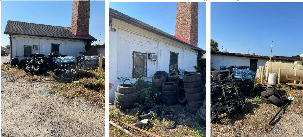
Figures 25-27: Stacked tires and empty water containers on the exterior of the office building
